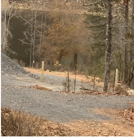
December 5, 2021 prior to gate construction
